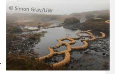
imported coir logs made of coconut fibre, with a future goal of lessening the carbon footprint of conservation works in Ireland.
